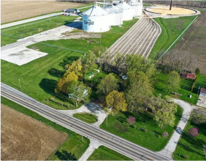
Cargill Grain Terminal - Tipton
