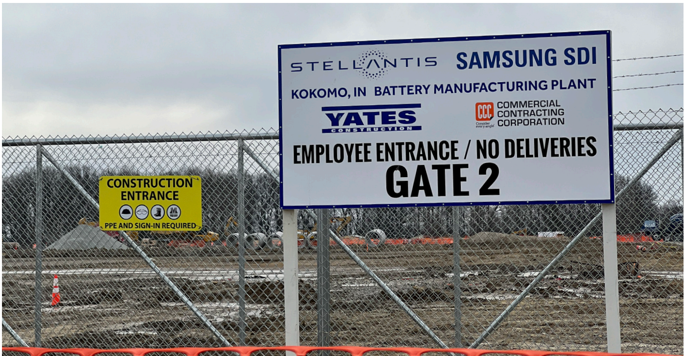
Stellantis/Samsung E.V. Plant Construction - Kokomo, IN
