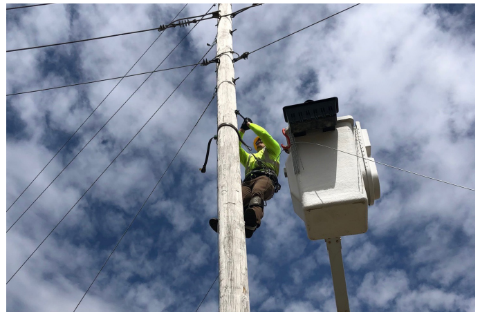
Fiber Installation - Cass County
